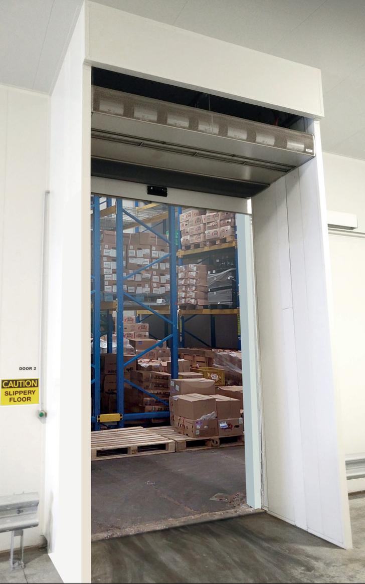
TRIOJET air curtain system is specially designed for freezers with large temperature differences. Ice, snow and fog are reduced, decreasing the risk of accidents while increasing energy savings and correct preservation of frozen products.
