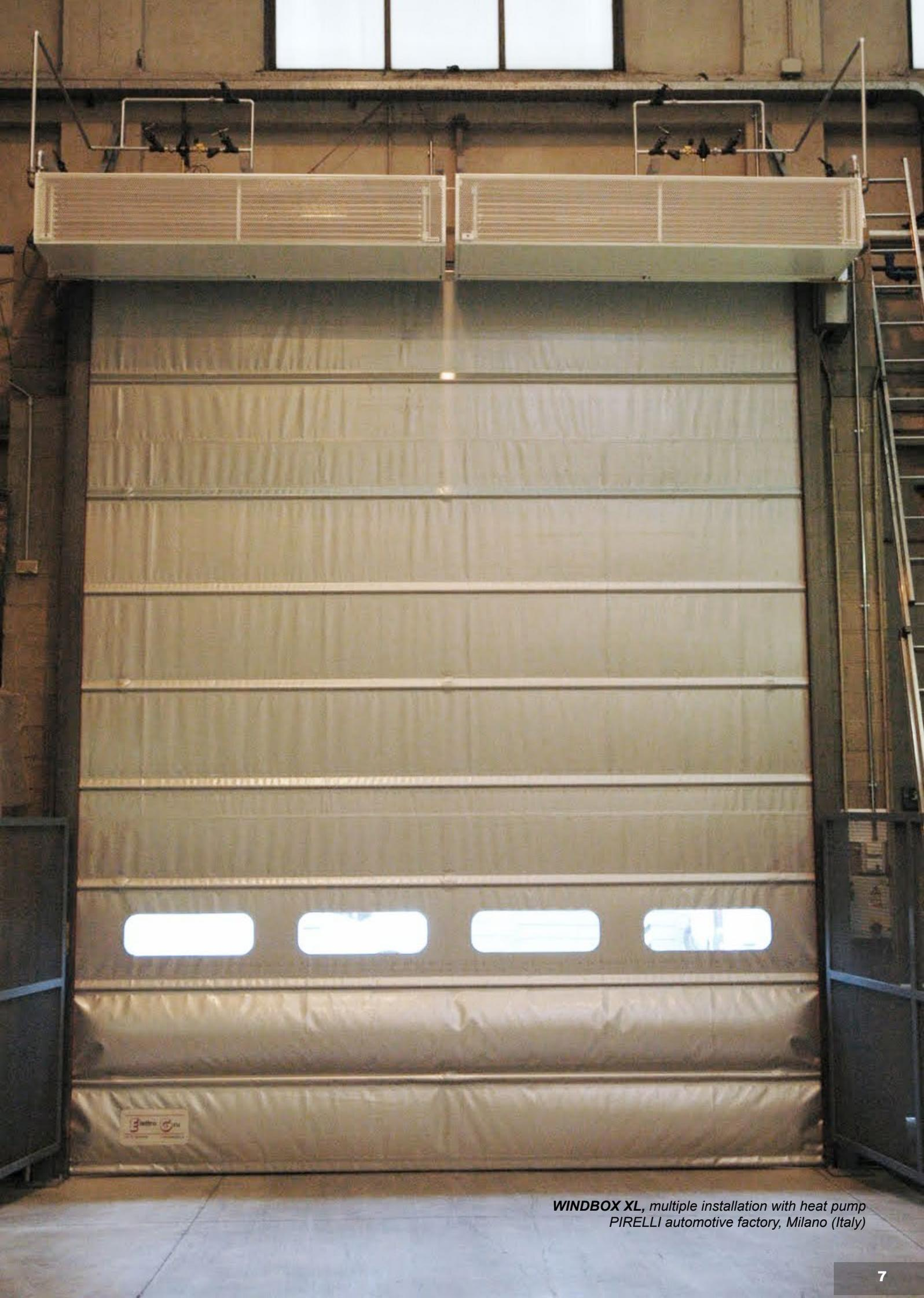
**WINDBOX XL**, multiple installation with heat pump
