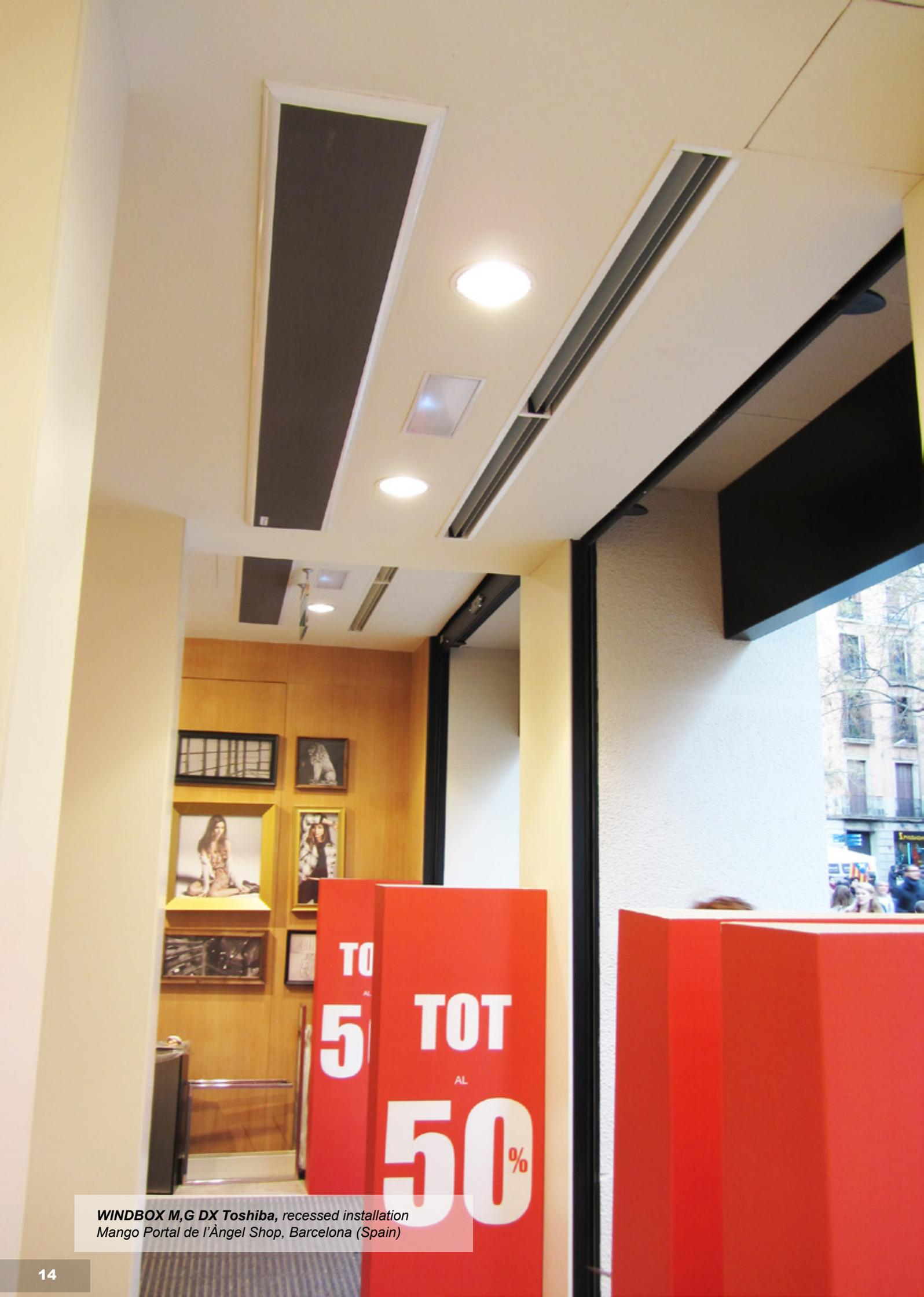
**WINDBOX M,G DX Toshiba**, recessed installation
